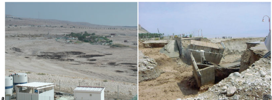
a collapse sinkhole field near a beach resort; b collapse of a bridge following a flood as a result of a headcut backward migration along the stream channel, demonstrating the effect of a powerful flood that was caused by the widening of the stream channel
