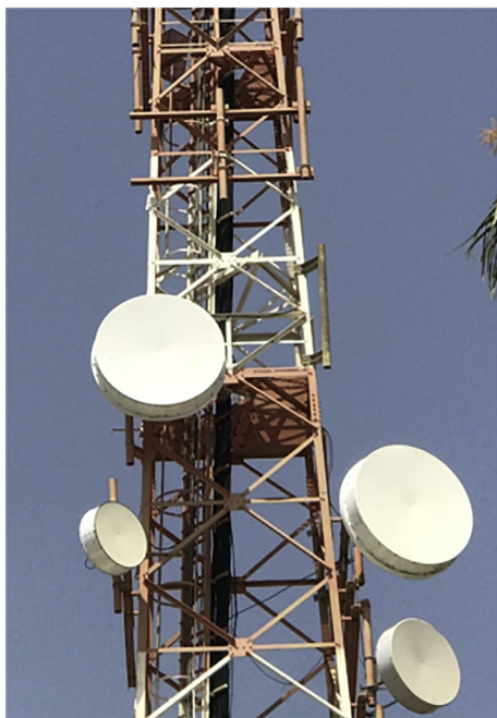
Fig. 1. A microwave communication mast.
