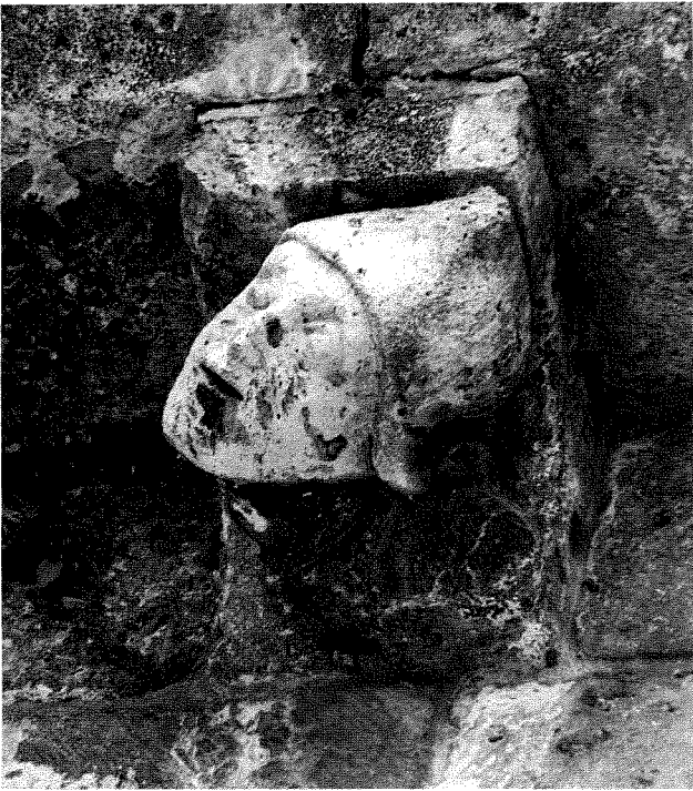
FIGURE 14. Moissac, Saint-Pierre, south facade: hooded male head (photo: author).
