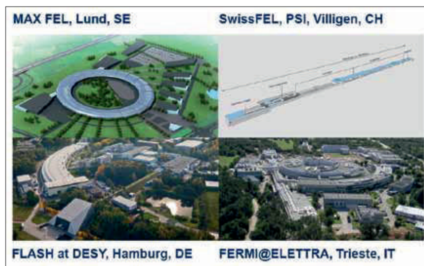
The first two operational X-ray FELs of EuroFEL in Germany and Italy and two advanced projects in Switzerland and Sweden (Copyright: Maxlab, PSI, DESY, FERMI@ELETTRA, Crozzoli).
