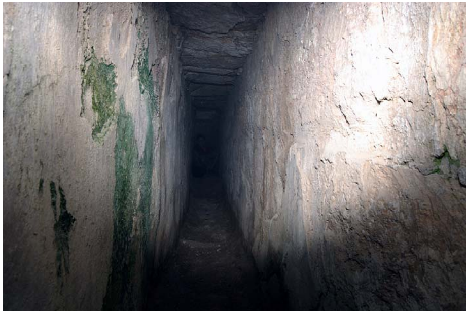
Fig. 11 – A Picture inside Tunnel A
