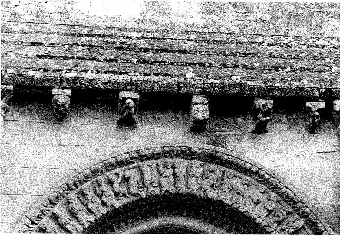
FIG. 1. Foussais, St. Hilaire, west facade, the corbel series
