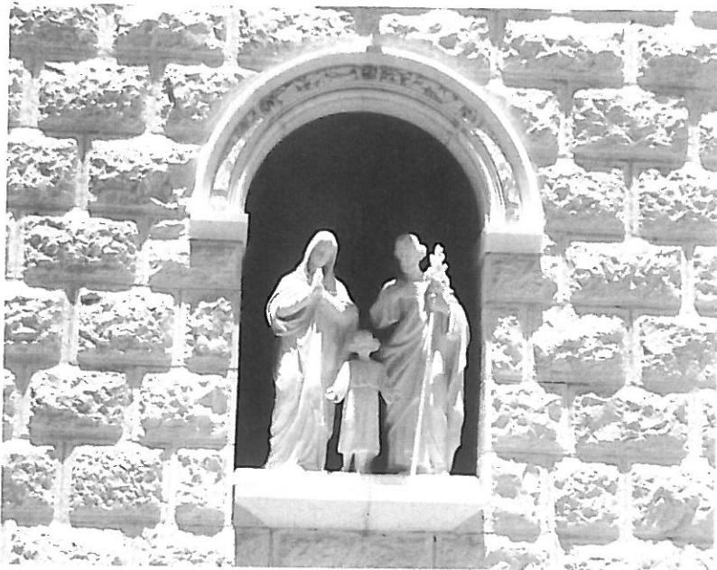
Fig. 4: Church of Saint Joseph Sculpture of Holy Family the southern façade
